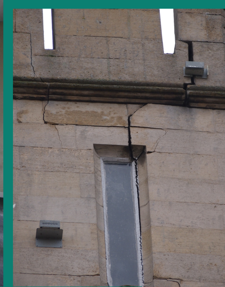
Cracks in tower and windows
