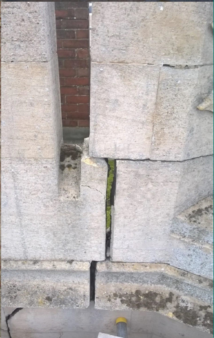
Cracks in tower and windows
